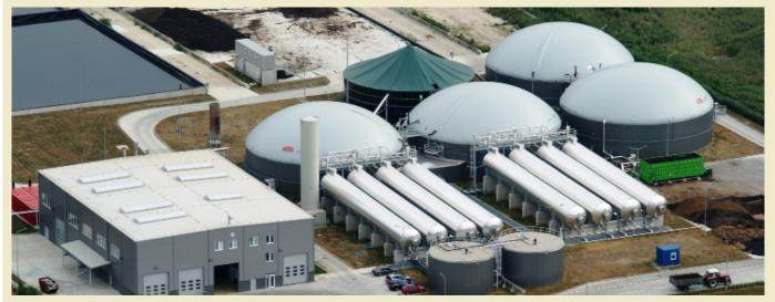
The biogas plant BOSANY is located 50km from Nitra (Slovakia). HEAT Bioenergy as a general contractor designed and built the complete plant on turn-key basis. The plant, which started its opertions in 2012, is designed to process approx. 100.000 t/y of organic residues and renewables, with an electric generation capacity of  $2 \times 1.4 \text{ MW}$ .
